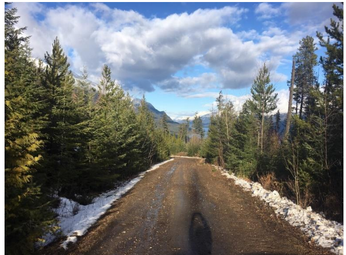
Branch 7 mainline after brushing and grading
