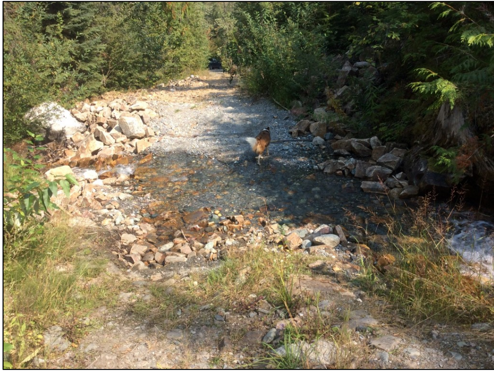
Image 9: View looking down at the second location where the diverted flow crosses the Bjerkness road (WP 96). The image shows the repairs to the road following the diversion of the flow down the road towards the Kaslo Back Road.
