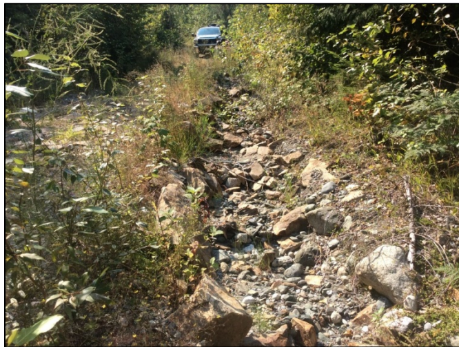
Image 8: View of the eroded channel forming a ditch as a result of the diverted flow (WP 94).
