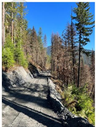
Sunshine Logging continues with the road construction into CP 52-1, with about 200m left before the end landing. Due to the amount of rock and steep switchbacks the road will require some earth moving to reduce the switchback grades and surface the rocky areas. With the temporary road construction the cut slopes are only 2-4 tall, significantly reducing the amount of time to construct the road.
