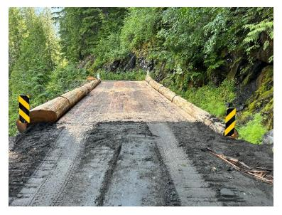
The bridge at 3km on Keen Creek was fixed by CJ Logging. It took more work than expected, including adding a stringer and some ties, as well as replacing the decking and curbs. It's ready for hauling now.
