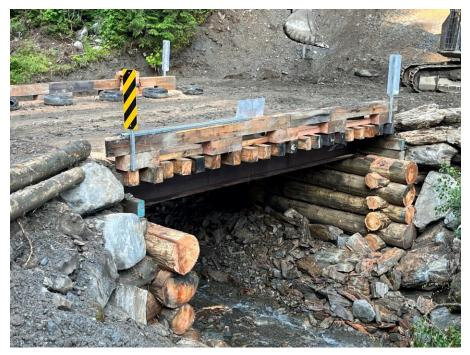
The bridge over Lost Ledge Creek is almost done, with about a week of work remaining. It was a tight crossing and blue clay was discovered in the cut slope banks trying to widen the road so the bridge had to be moved slightly and extra work done to ensure the stability of the site. The bridge is being certified by the designer, SNT from Nelson, in accordance with professional standards.
